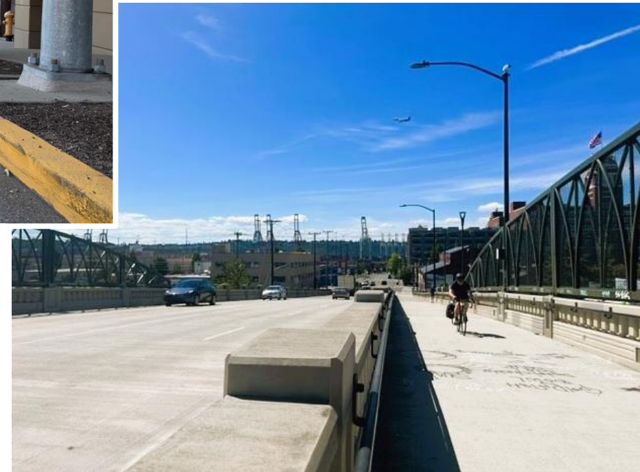
Top: John Lewis Memorial Bridge Bottom: Lander St Bridge
