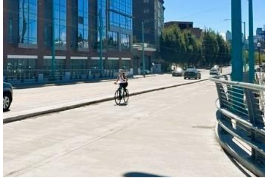
Top to bottom: Fairview Ave N Bridge, with two-way PBL; Repaving on E Madison St as part of Madison RapidRide G Line project; Repaved SW Avalon Way with new PBL.
